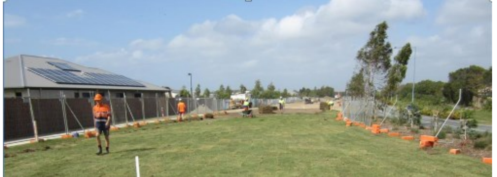
Grass areas are currently being restored, after extensive Pipeline Construction works.
